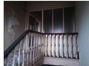
YARM LANE - SECOND FLOOR STAIR LANDING
