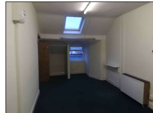
YARM LANE - SECOND FLOOR TYPICAL ROOM
