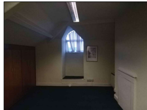
YARM LANE - SECOND FLOOR DORMER WINDOW
