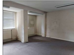
BARRINGTON HOUSE - REAR TWO-STOREY EXTENSION TO BOWLSFIELD LANE
